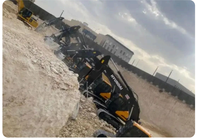
Rock cutting and profiling of excavation slopes
