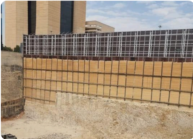
Shoring to a deep excavation adjacent to existing towers, Riyadh
