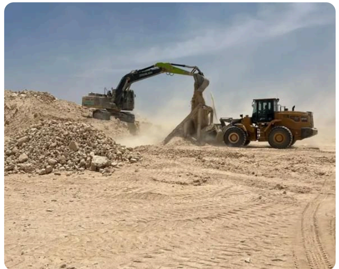
Loading and haulage of demolition arisings
