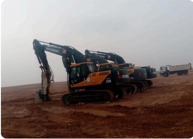
Excavation, levelling and haulage of excavated material
