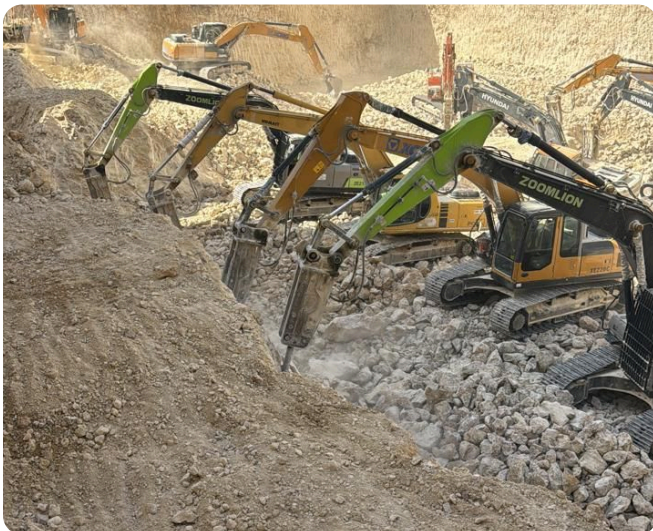
Rock breaking adjacent to existing structures
